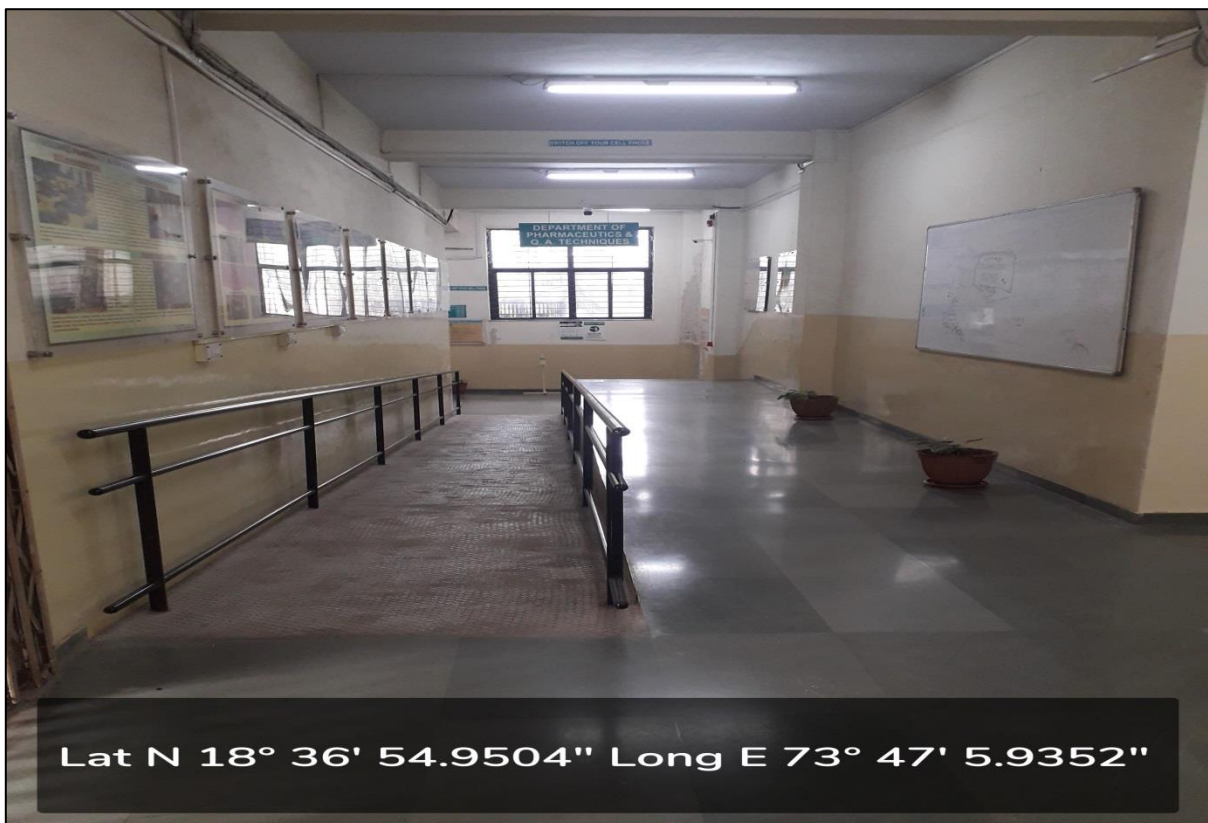
Availability of ramp for barrier free entry
